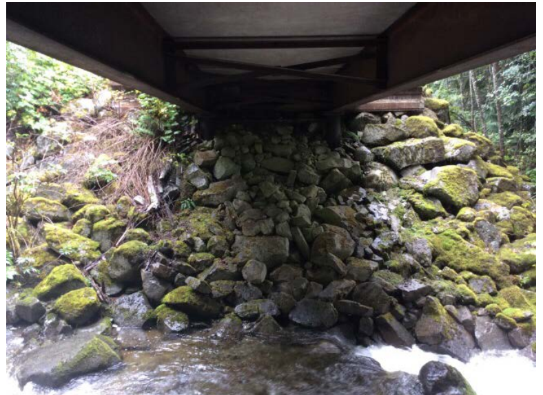
Left Bank Abutment when facing downstream
